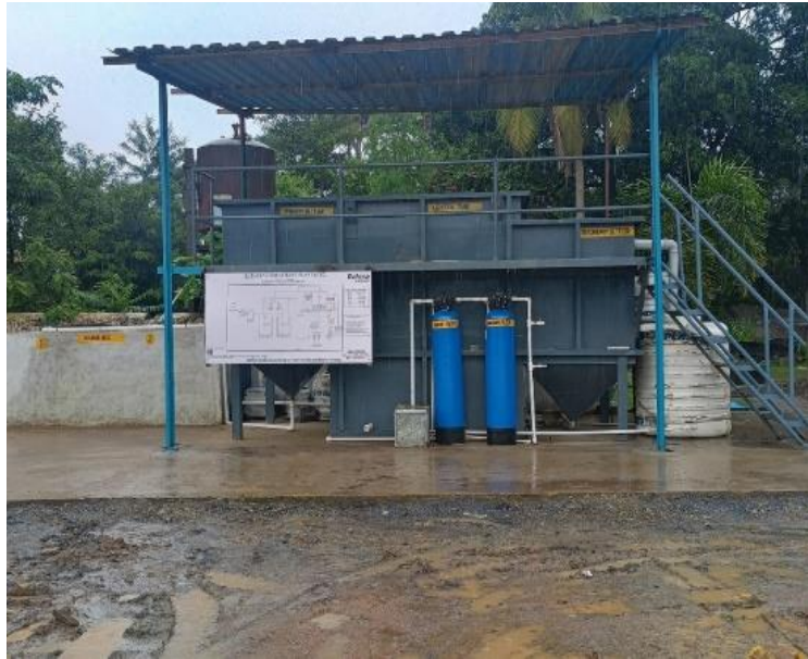
ETP of Capacity 25 KLD
