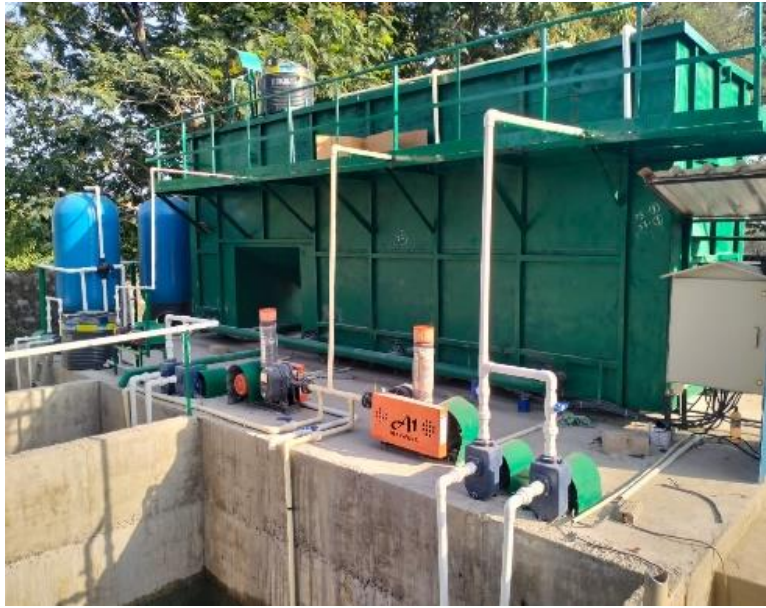
STP of Capacity 75 KLD
